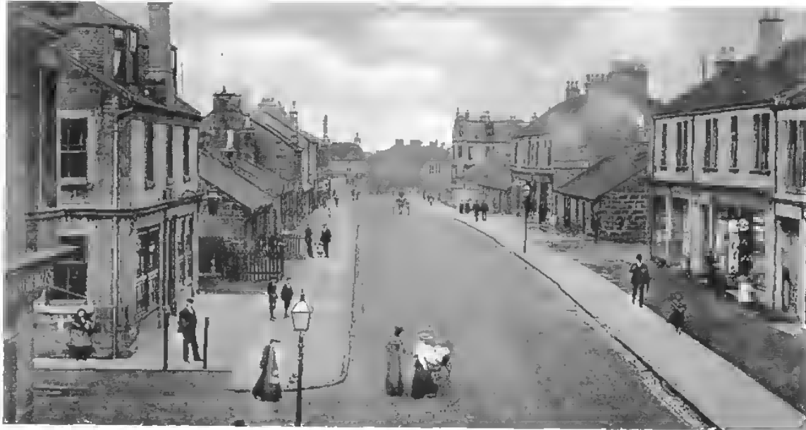
1890s HAMILTON ROAD AGAIN, FROM THE CROSS ON THE RIGHT
